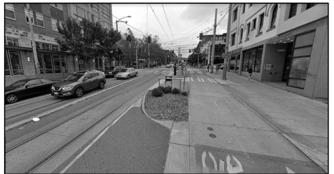
Figure 1 Before and after example of a road safety project: installation of two-way protected bike lanes and a road diet on Broadway in Seattle's Capitol Hill neighbourhood. Source: Google Street View.
