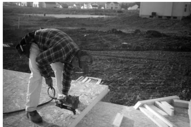
Figure 1 Contact trip stapler gun.
