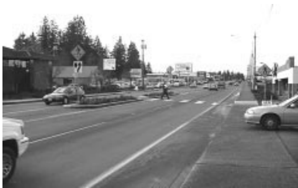
Figure 1 Photograph of a pedestrian refuge island in a busy four lane arterial highway.
